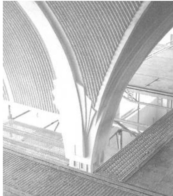
**Fig. 9** Arches and ceilings with a mortar cover in comb form with dangerous sound absorption for high frequencies
